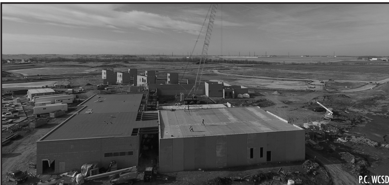
Construction on Waukee’s Trailridge School as of February 2022.
